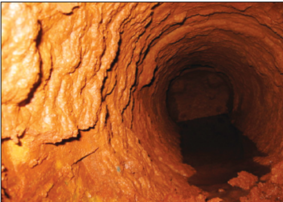
Figure 1. Iron mineral precipitation in a water distribution system.
